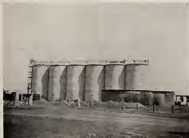
NEW CONCRETE TANKS AT LOCKHART, N. S. W.
